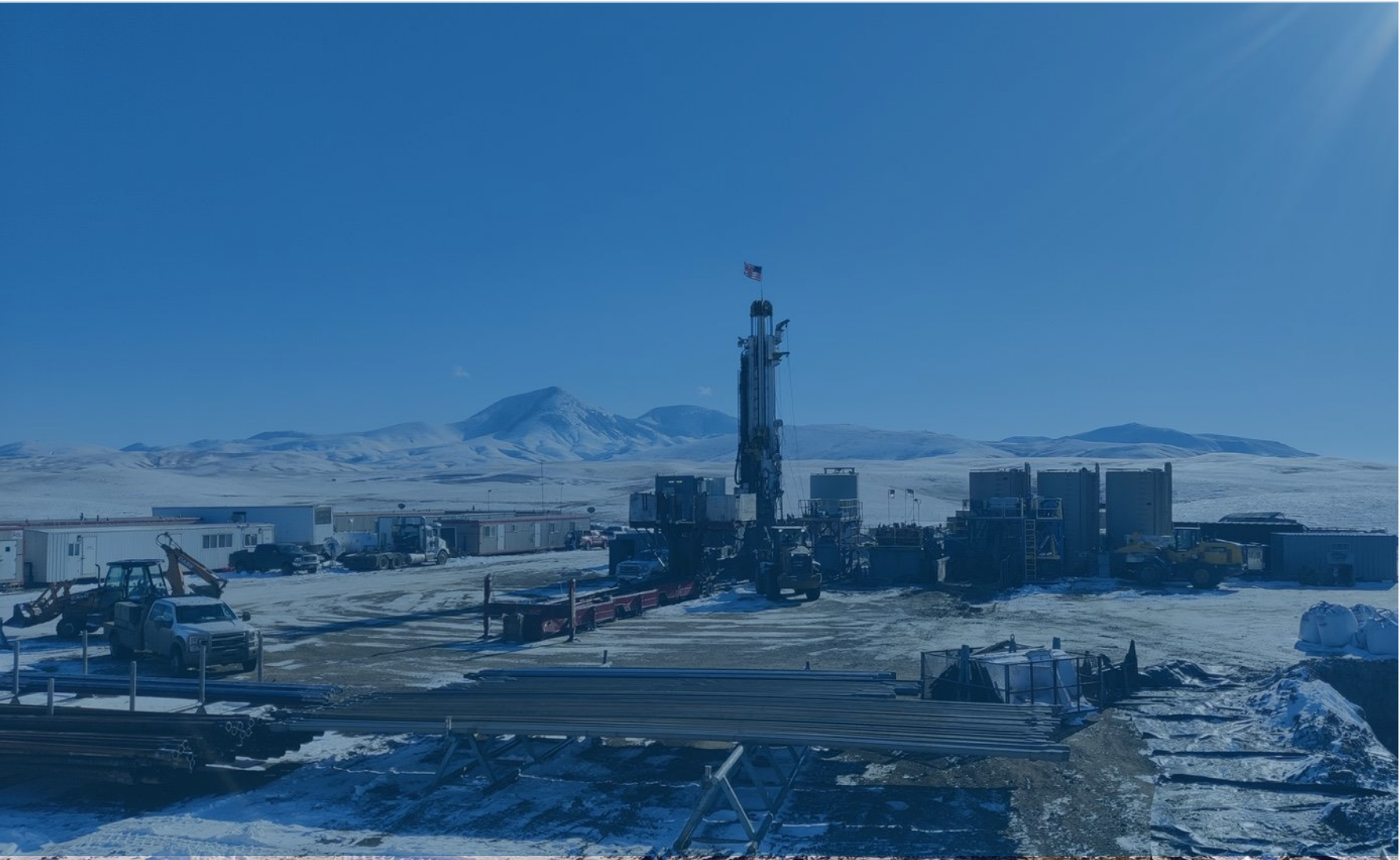
Avanti’s WNG 10-21 Well during drilling
